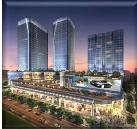
Shanghai Cullinan (ICC Residence)
