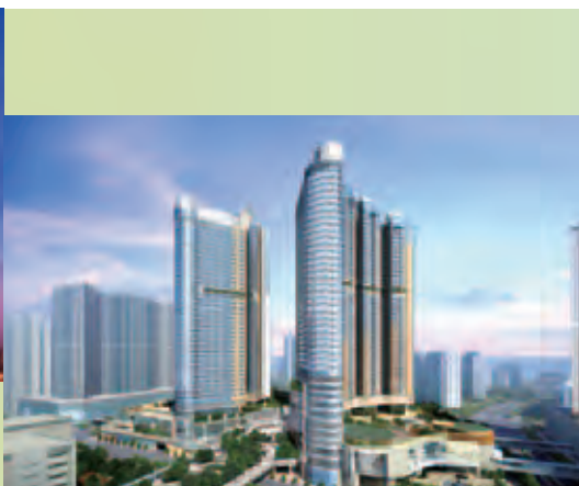
將軍澳港鐵站上蓋綜合發展項目 Integrated complex atop Tseung Kwan O Station
